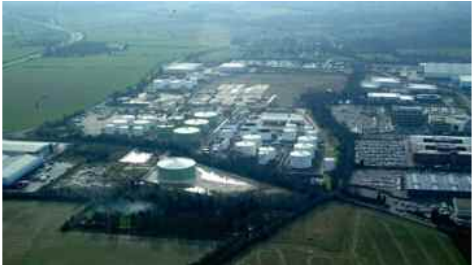
Figure 7 The area prior to incident
