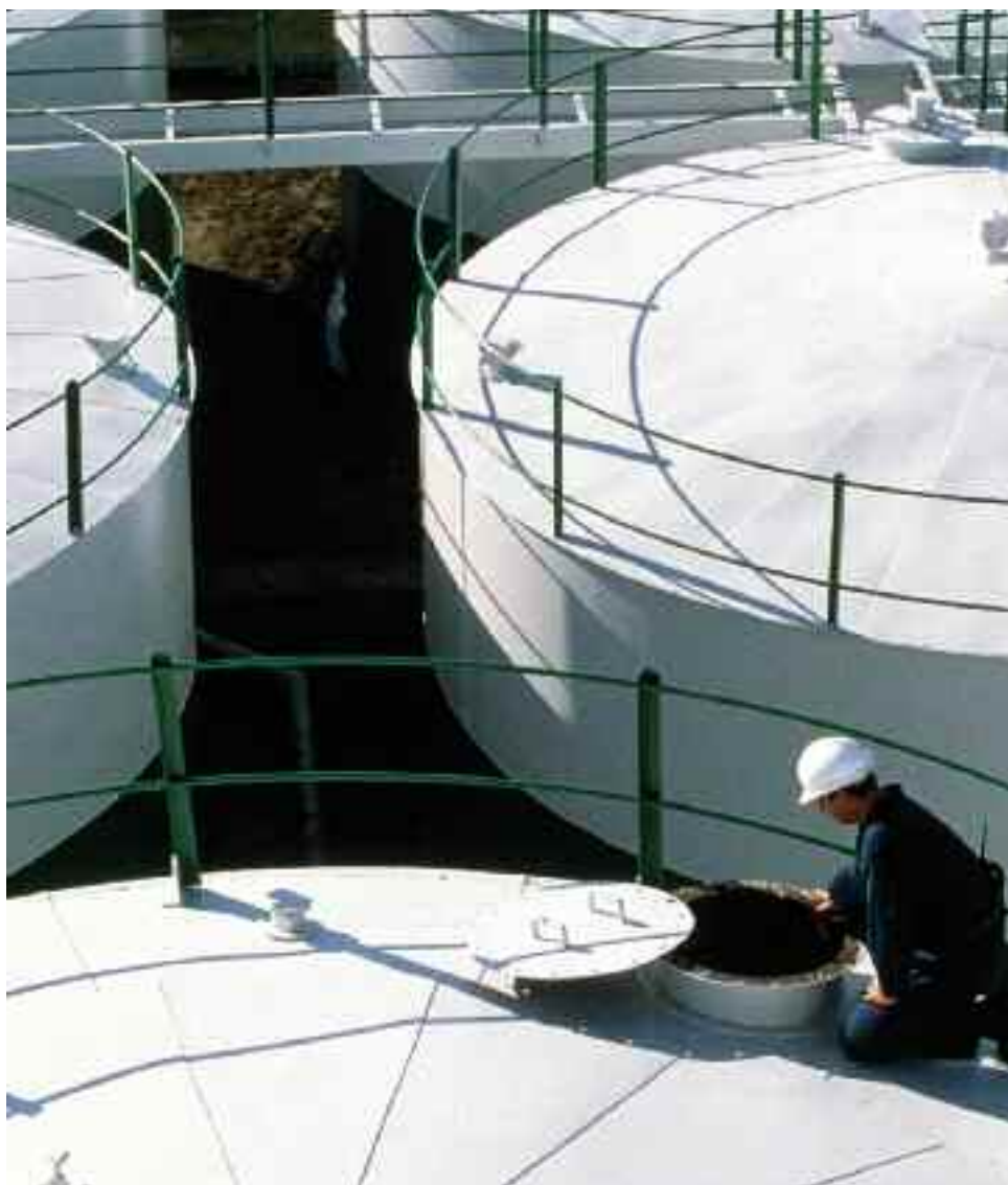
Figure 10 Maintenance worker inspecting a tank top
