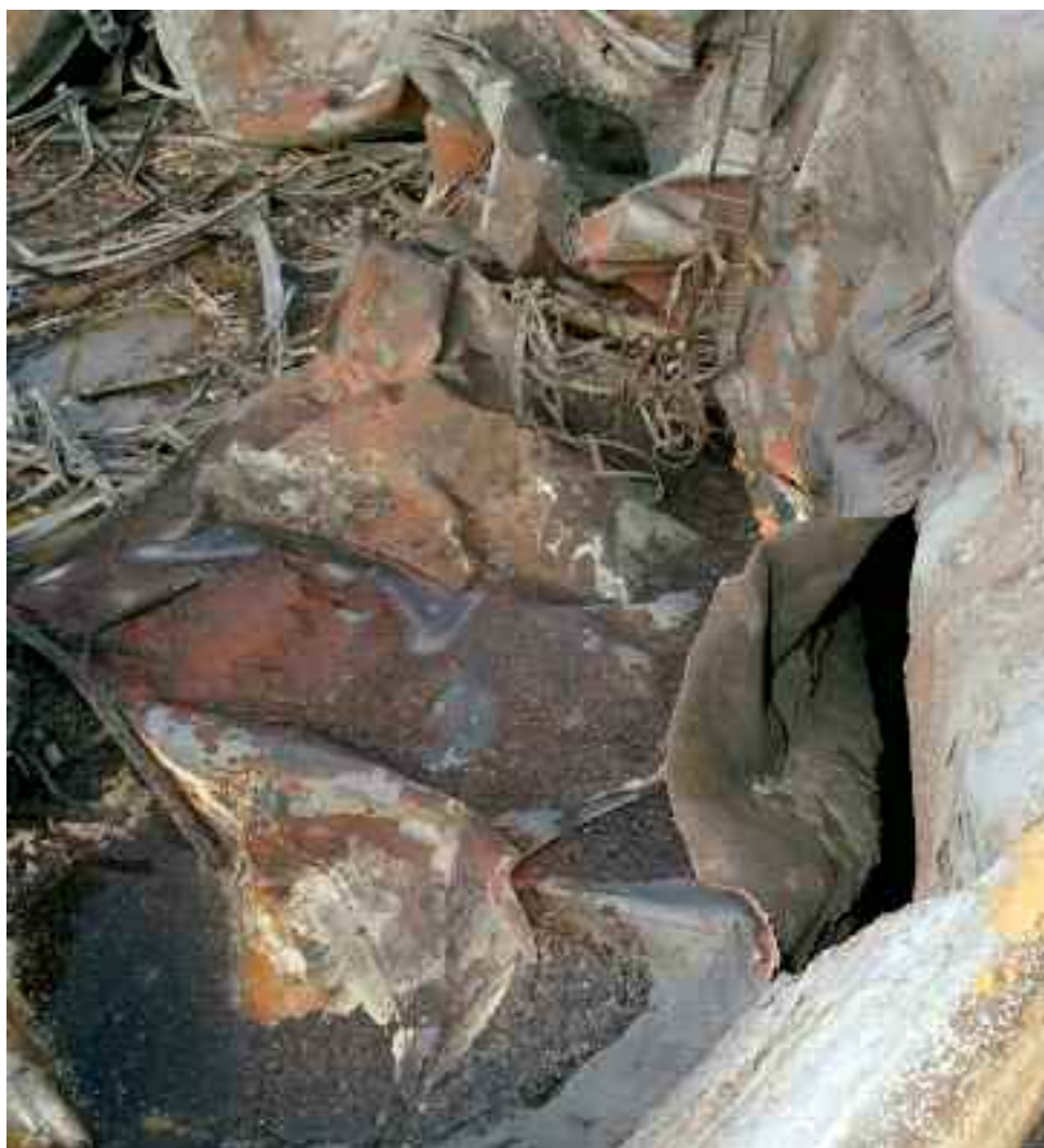
Figure 9 View into Tank 912
