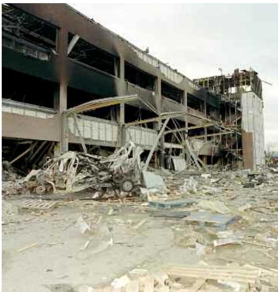
Figure 5 North side of the Northgate building
